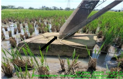
Gambar 3. Kabel Ground wire
