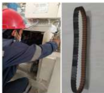
Gambar 4. Pergantian Timming Belt 1422 V255 .
