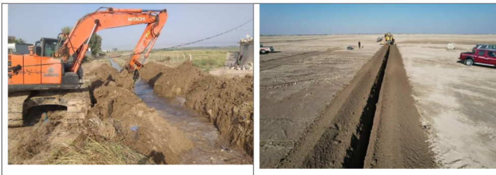
Figure 4. Early Stages of Construction and Earthwork: Excavation and Smoothing
