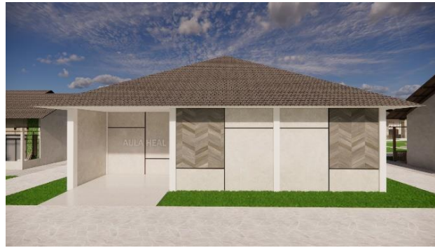
Figure 8. Façade of the Hall Building
