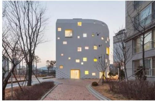
Figure 3: Building of Flower + Kindergarten / OA-Lab
