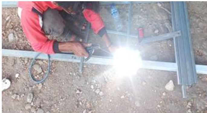
Gambar 6 Proses Pengelasan Besi Hollow
